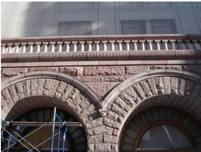
Figure 1. The American Museum of Natural History in New York City chose natural cement repointing mortar, replicating the original 1892 material, consciously embracing Authenticity and preserving the building's historic integrity.
