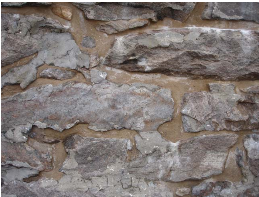
Figure 5. Natural cement mortar saves labor costs by allowing single-lift build-out, regardless of joint width and depth.
