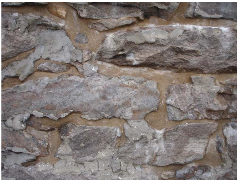
Figure 5. Natural cement mortar saves labor costs by allowing single-lift build-out, regardless of joint width and depth.
